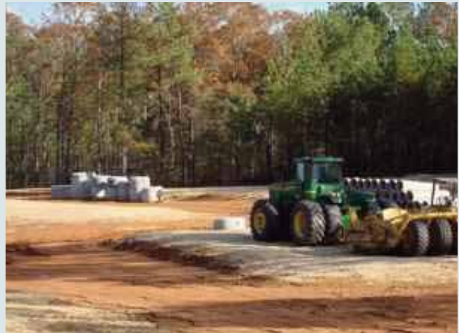
Storm sewers stand ready to be installed.
