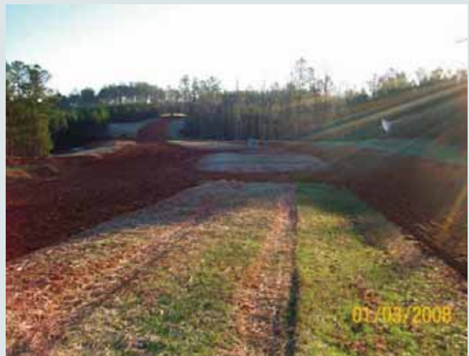
The community entrance begins to take shape.
