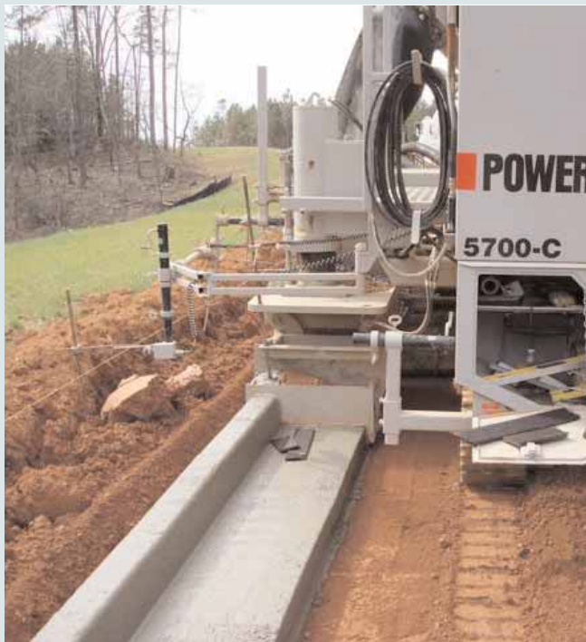
Curb construction is well underway.
