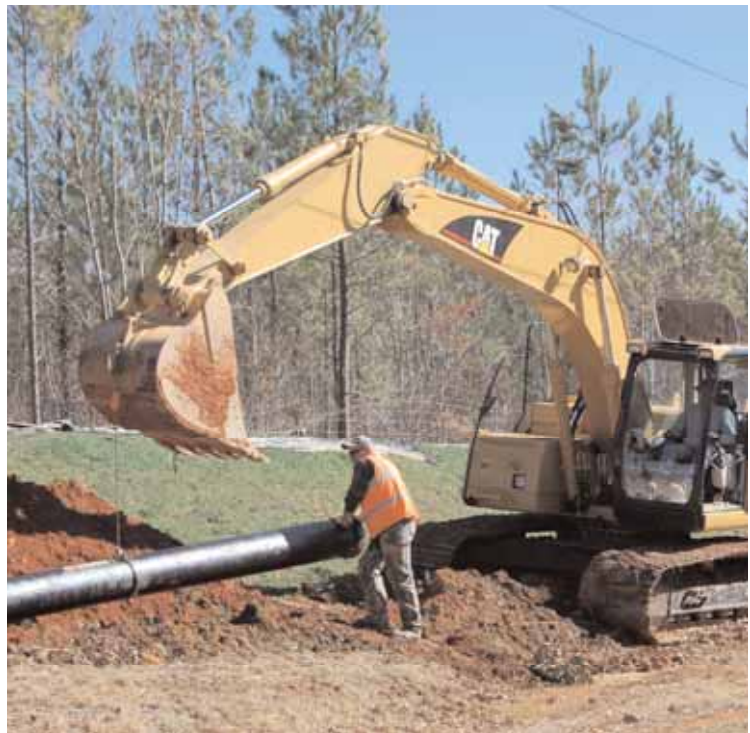
Water/sewer lines installation at the main entrance.
